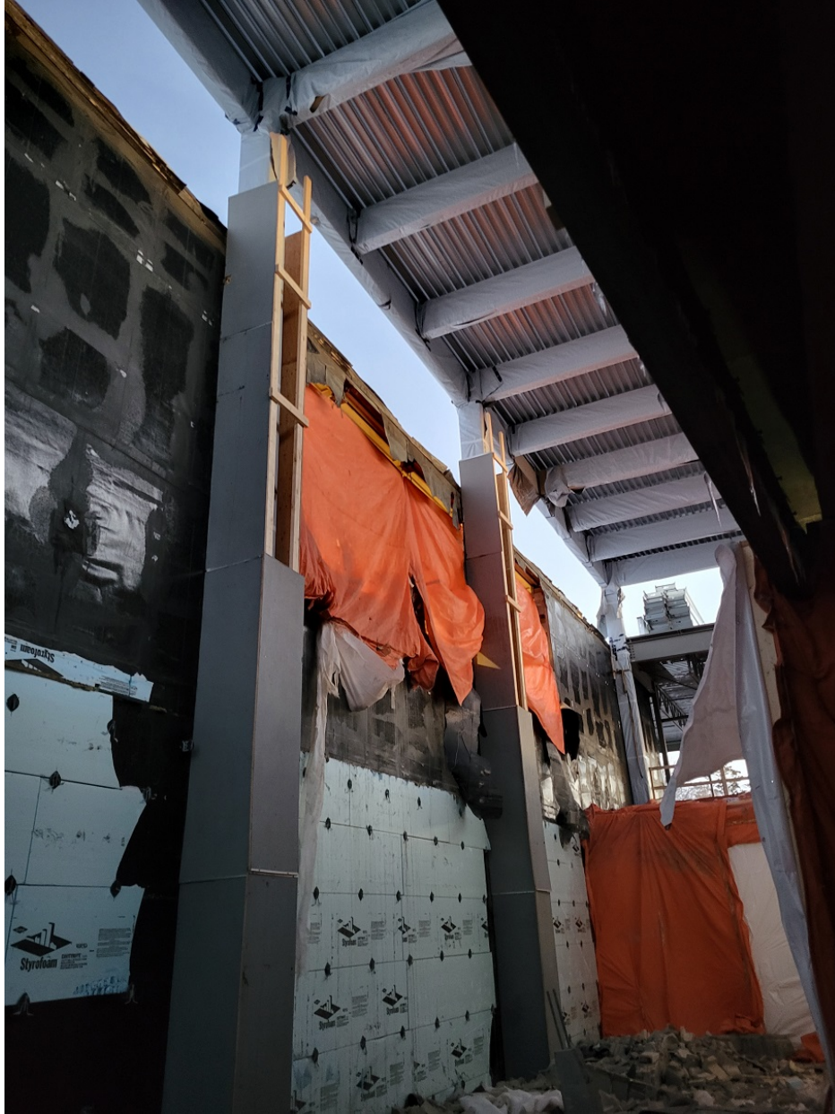
Photo #8 – Clerestory Protection and Roof Deck
