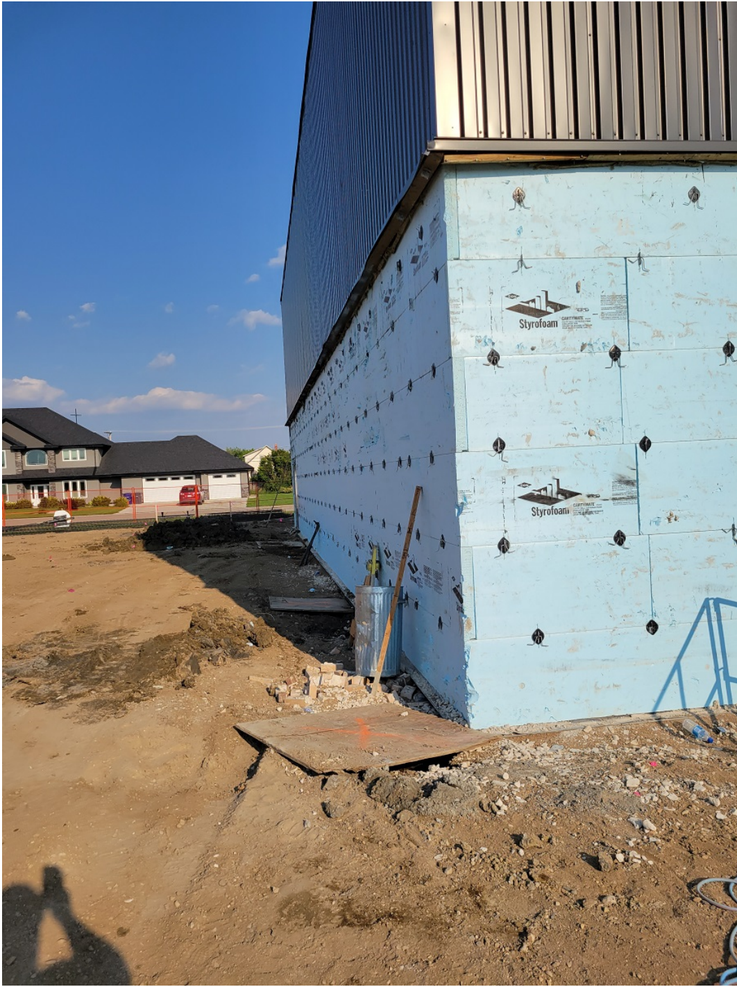
Photo #06 – North east corner of existing gym brick removed with piles covered.
