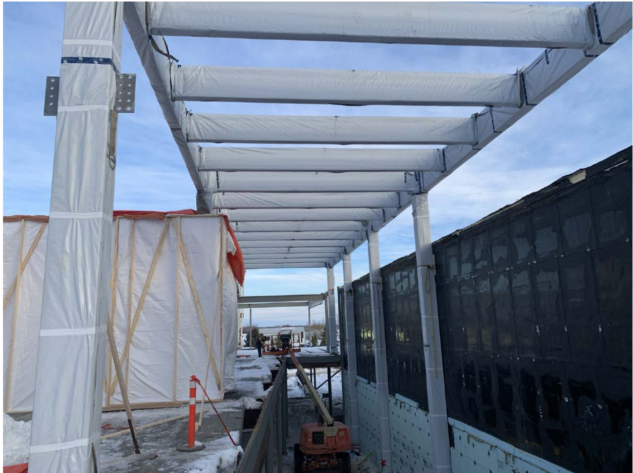
Photo #02 – Glulam installed
