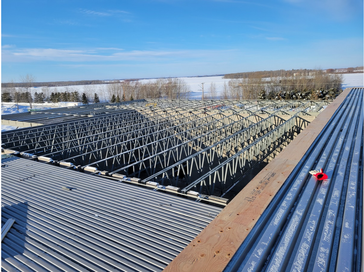
Photo #1 – Room 106 Trusses and Roof Decking
