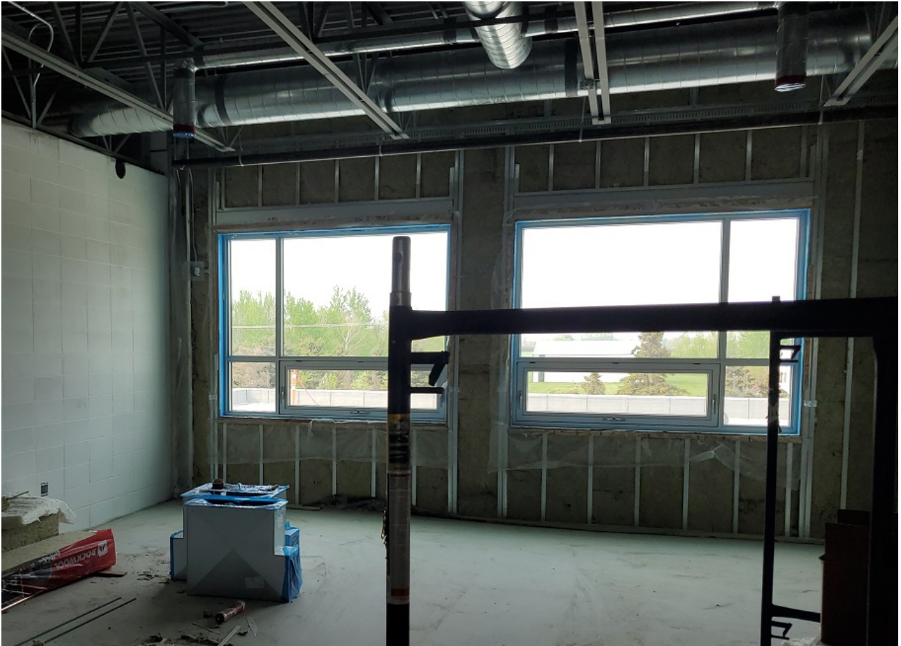
Photo #9 – Second Floor Classroom Exterior Wall Insulation
