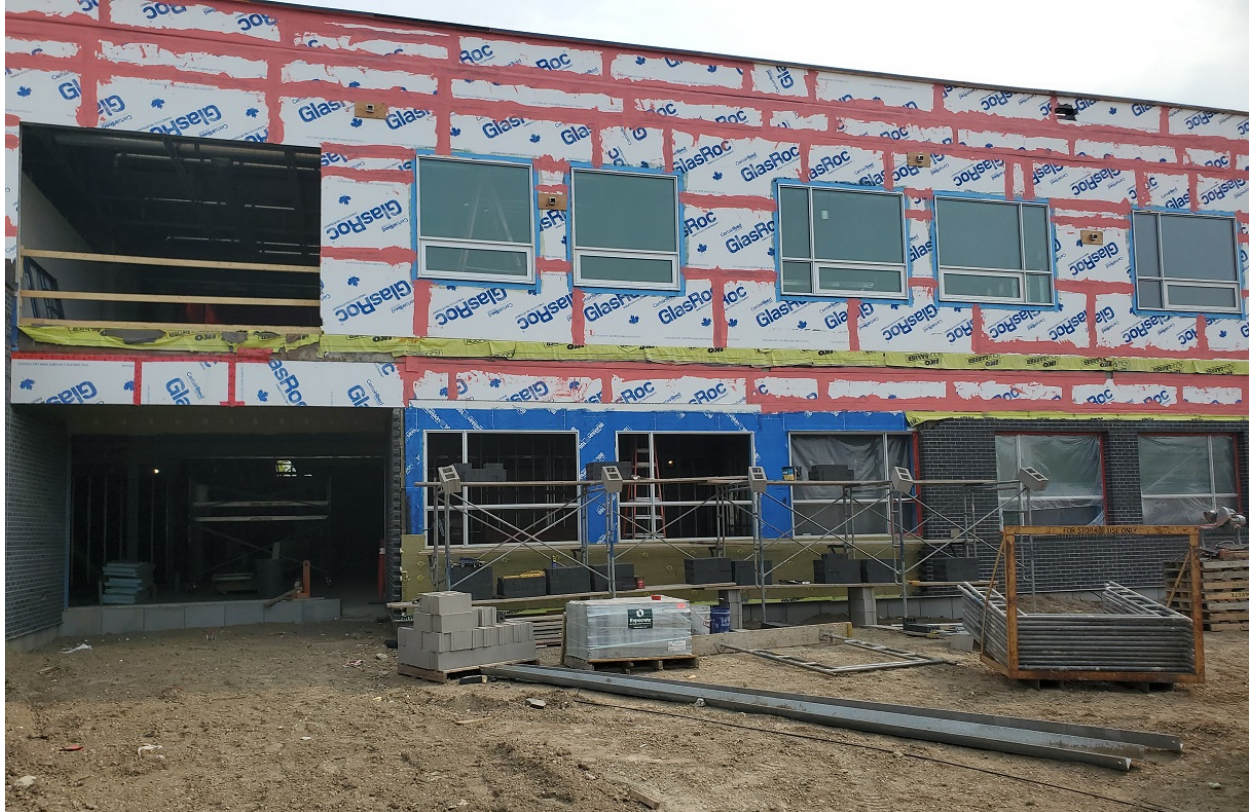
Photo #2 – Exterior EIFS Vapour Barrier
