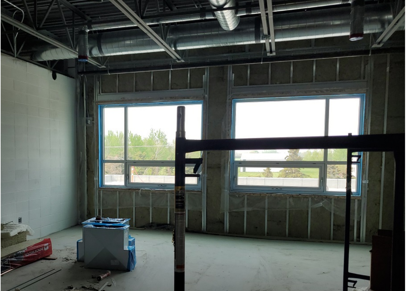
Photo #9 – Second Floor Classroom Exterior Wall Insulation
