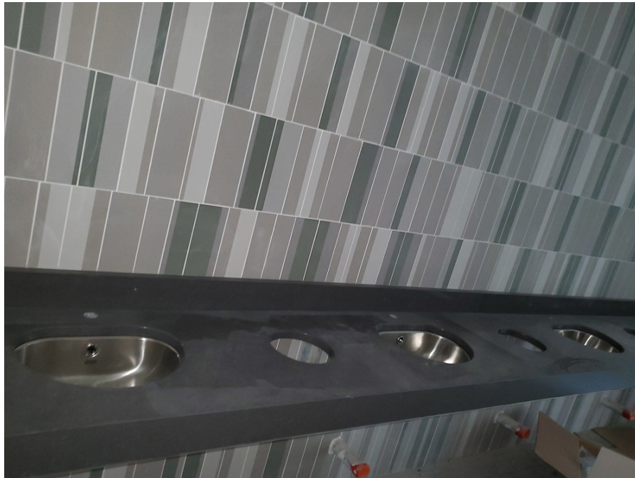
Photo #5 – Second Floor Washroom Area
