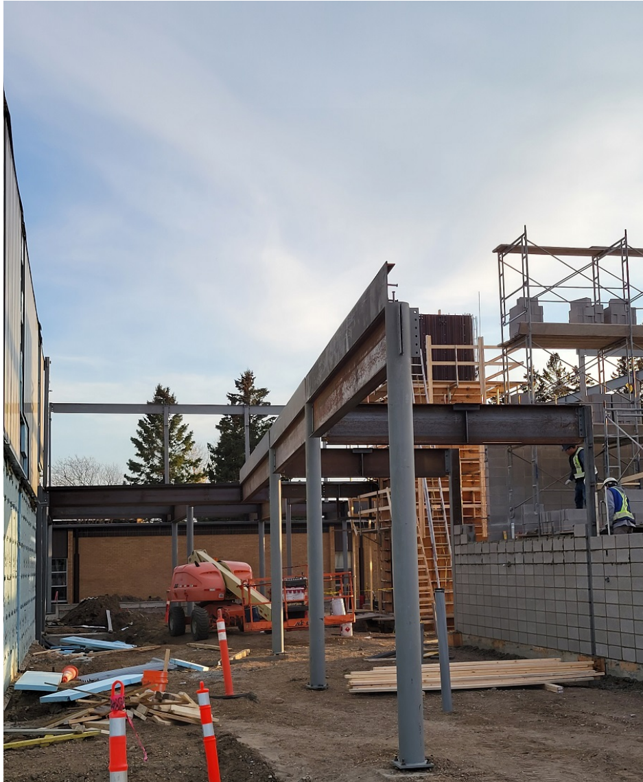
Photo #01 – Clerestory Area
