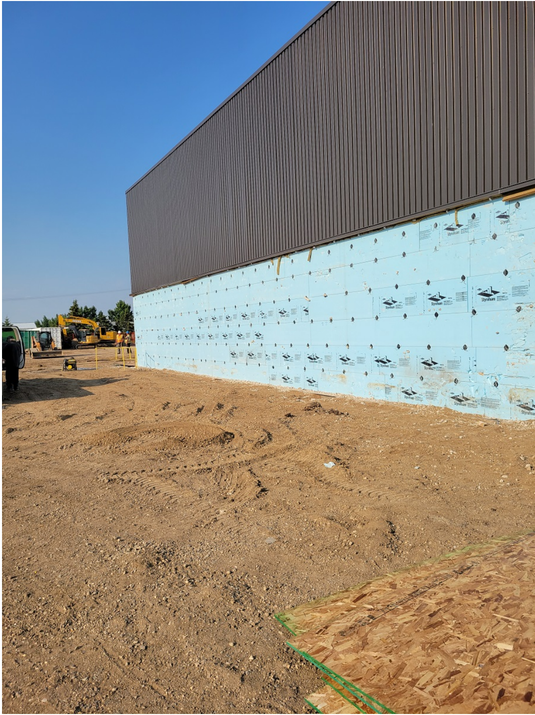
Photo #05 – West side of existing gym brick removed
