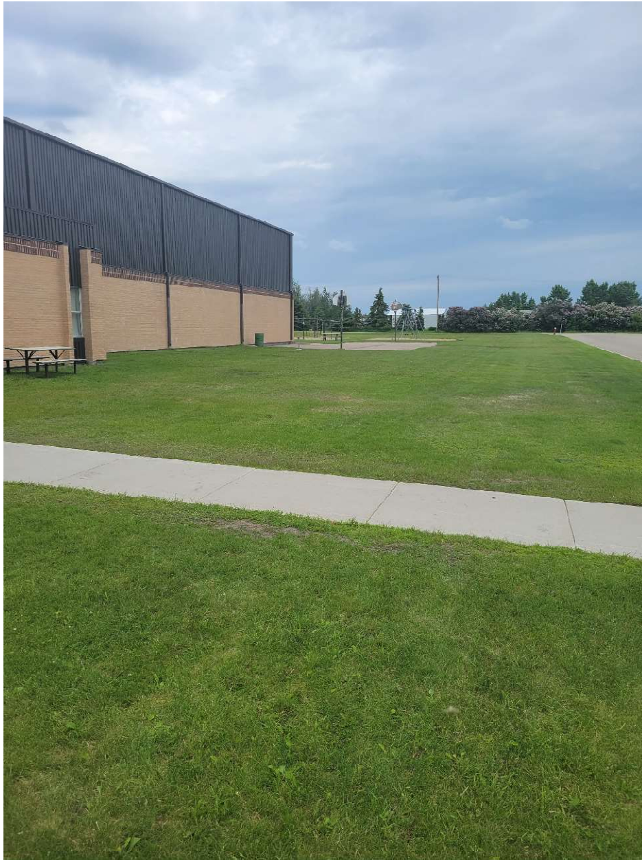
Photo #01 – Pre-Construction, East Side of Gym, Basketball Tarmac, Playgrounds
