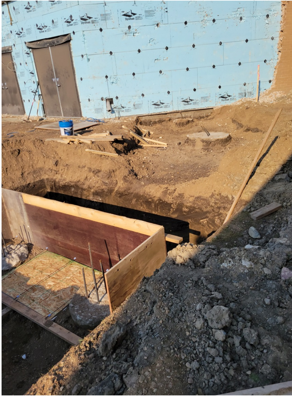
Photo #04 – Piles along Grid Line 2 at new main entrance to school
