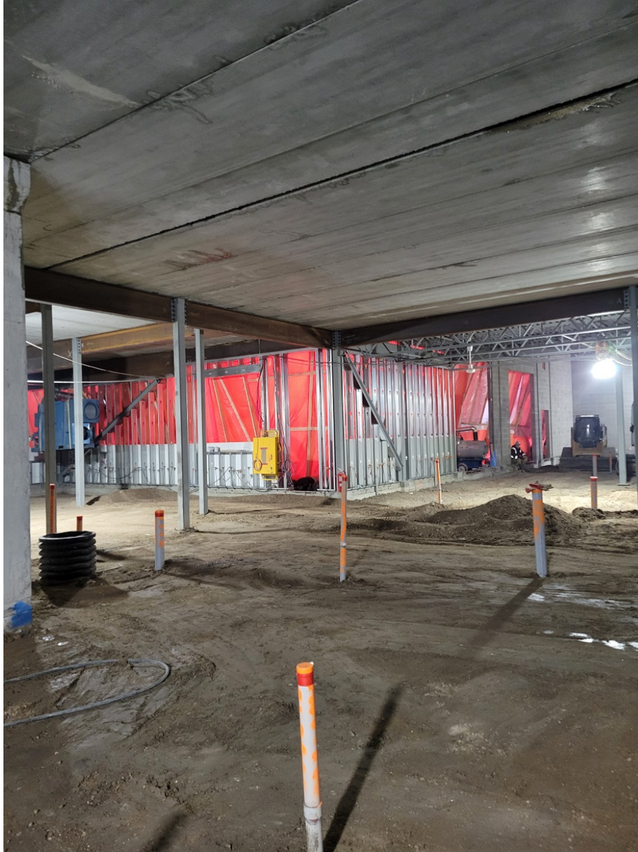
Photo #6 – Phase 1 Undergrounds for Slab Prep
