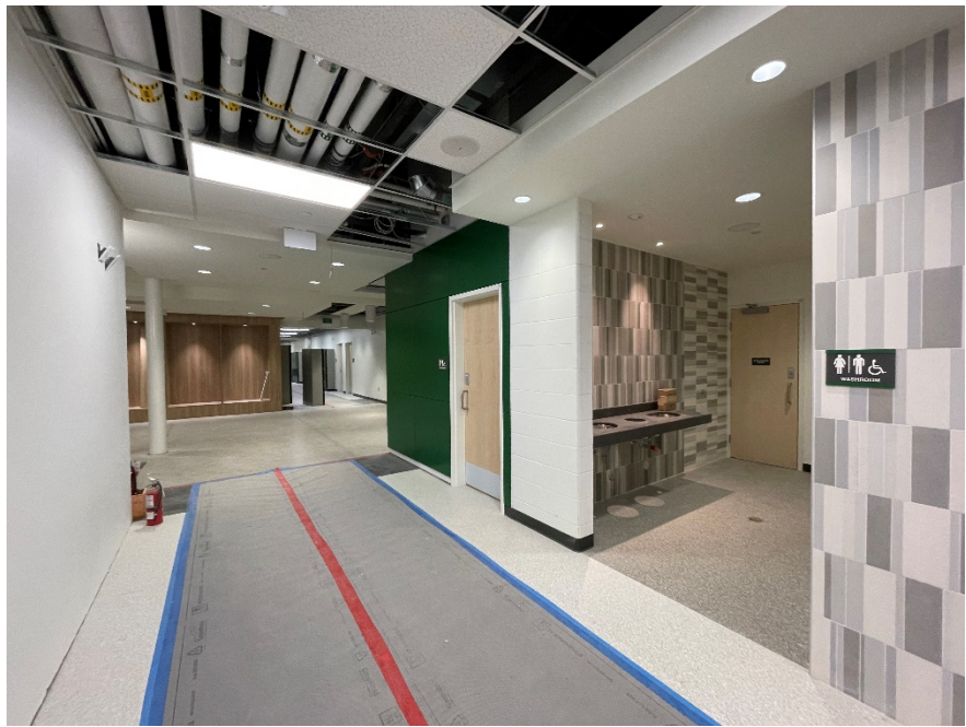
Photo #6 – First Floor Washroom Entrance
