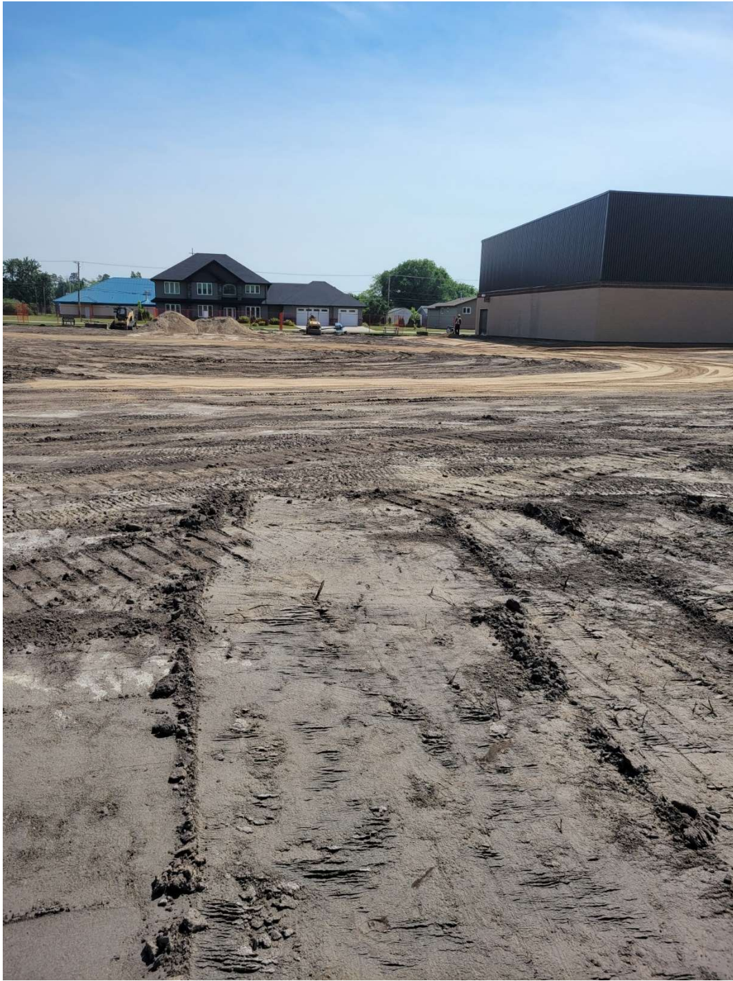
Photo #06 – Stripped Site
