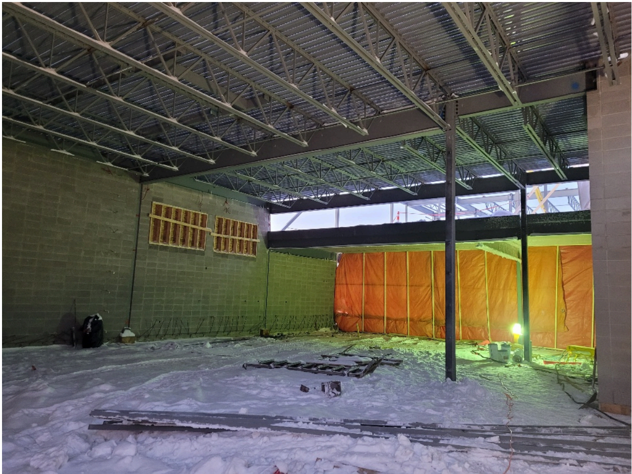
Photo #7 – PAA room looking north
