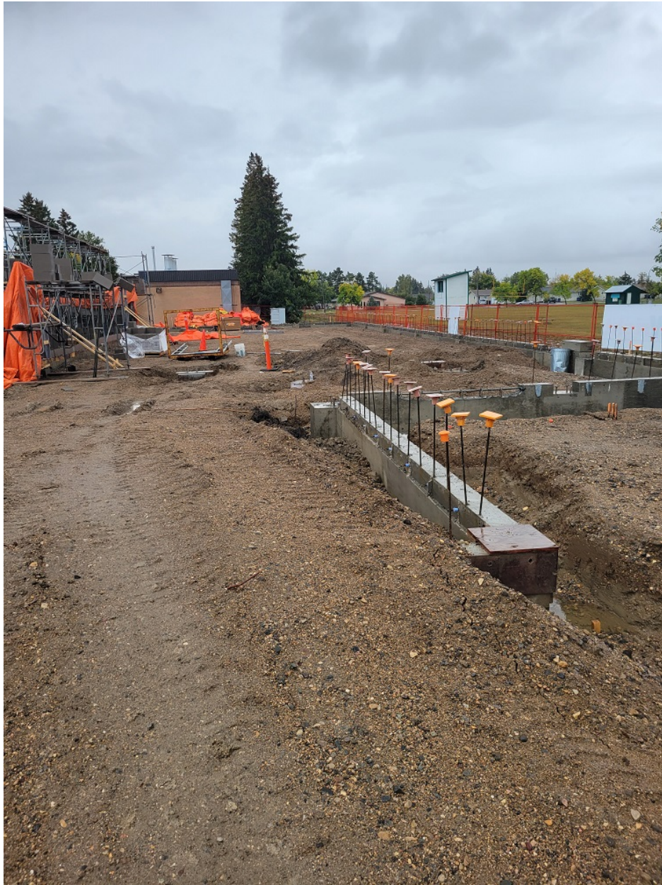
Photo #03 – Grade Beam along Grid Lines 8 & B looking south
