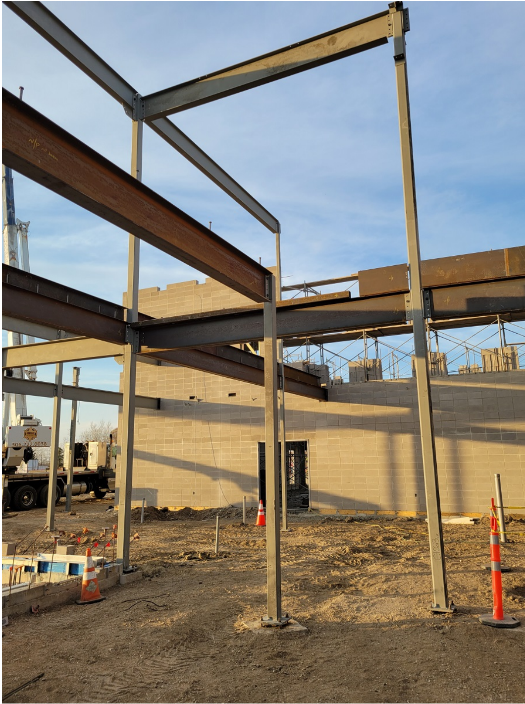
Photo #06 – Room 106 Masonry Steel
