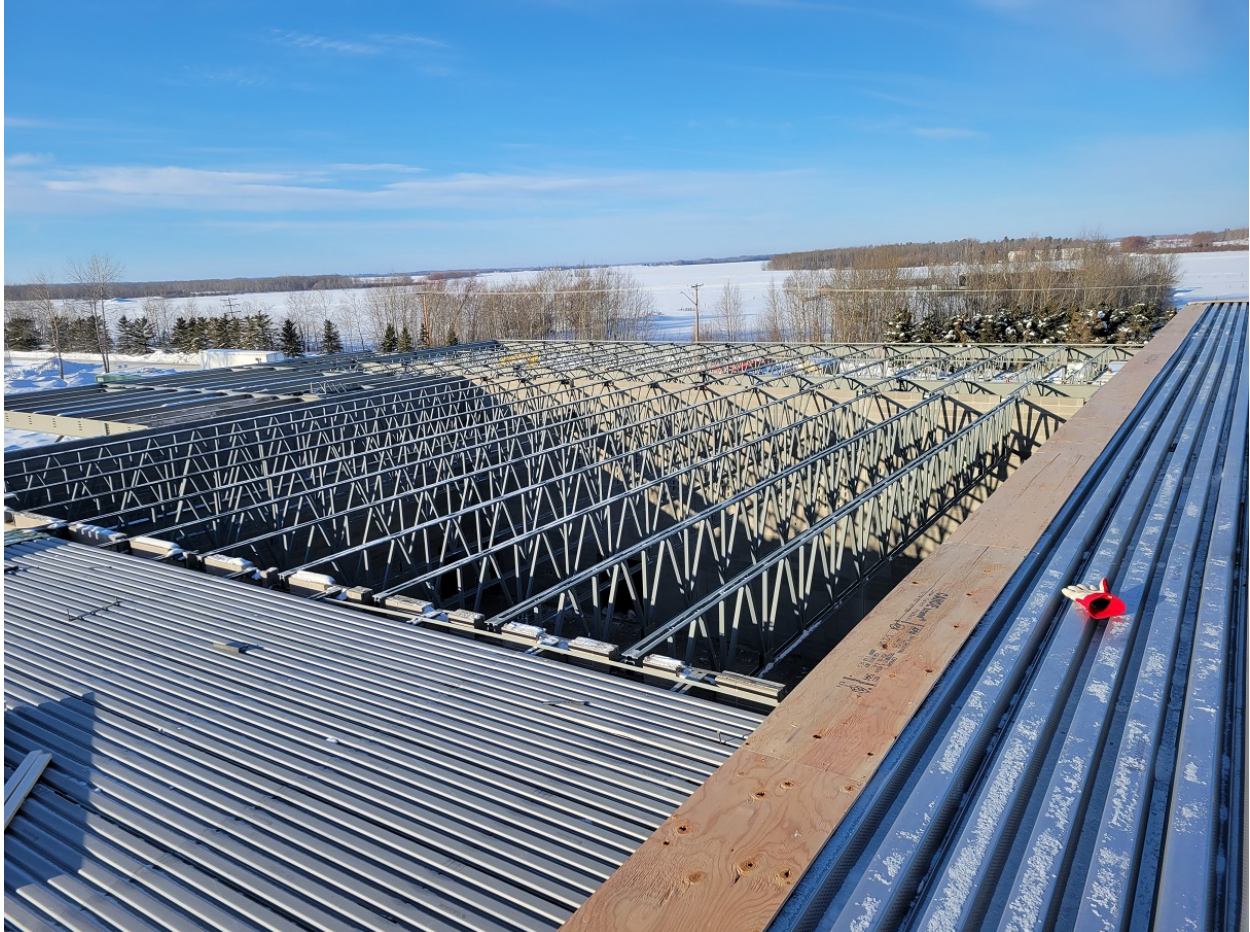
Photo #1 – Room 106 Trusses and Roof Decking
