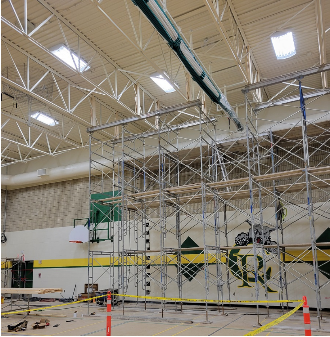
Photo #06 – Existing Gym Structural Scaffold
