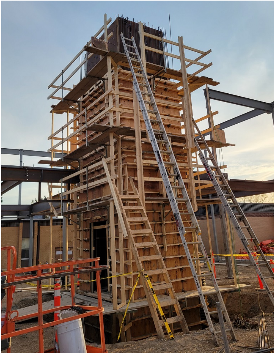
Photo #03 – Elevator Shaft
