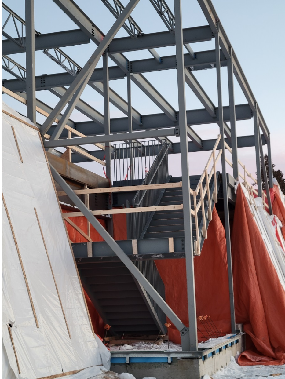
Photo #5 – Stairwell 4 in North West Corner
