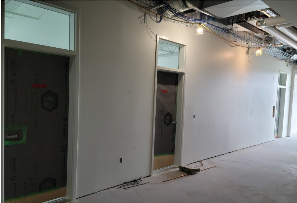
Photo #9 – Wood Doors
