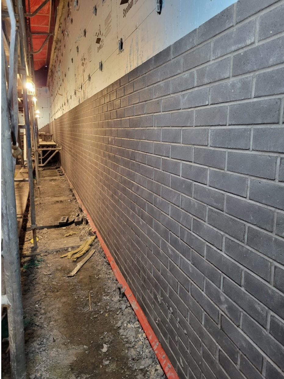
Photo #7 – Exterior Brick Veneer
