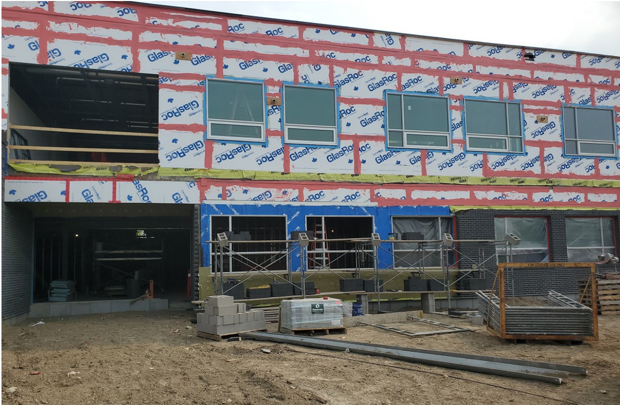
Photo #2 – Exterior EIFS Vapour Barrier
