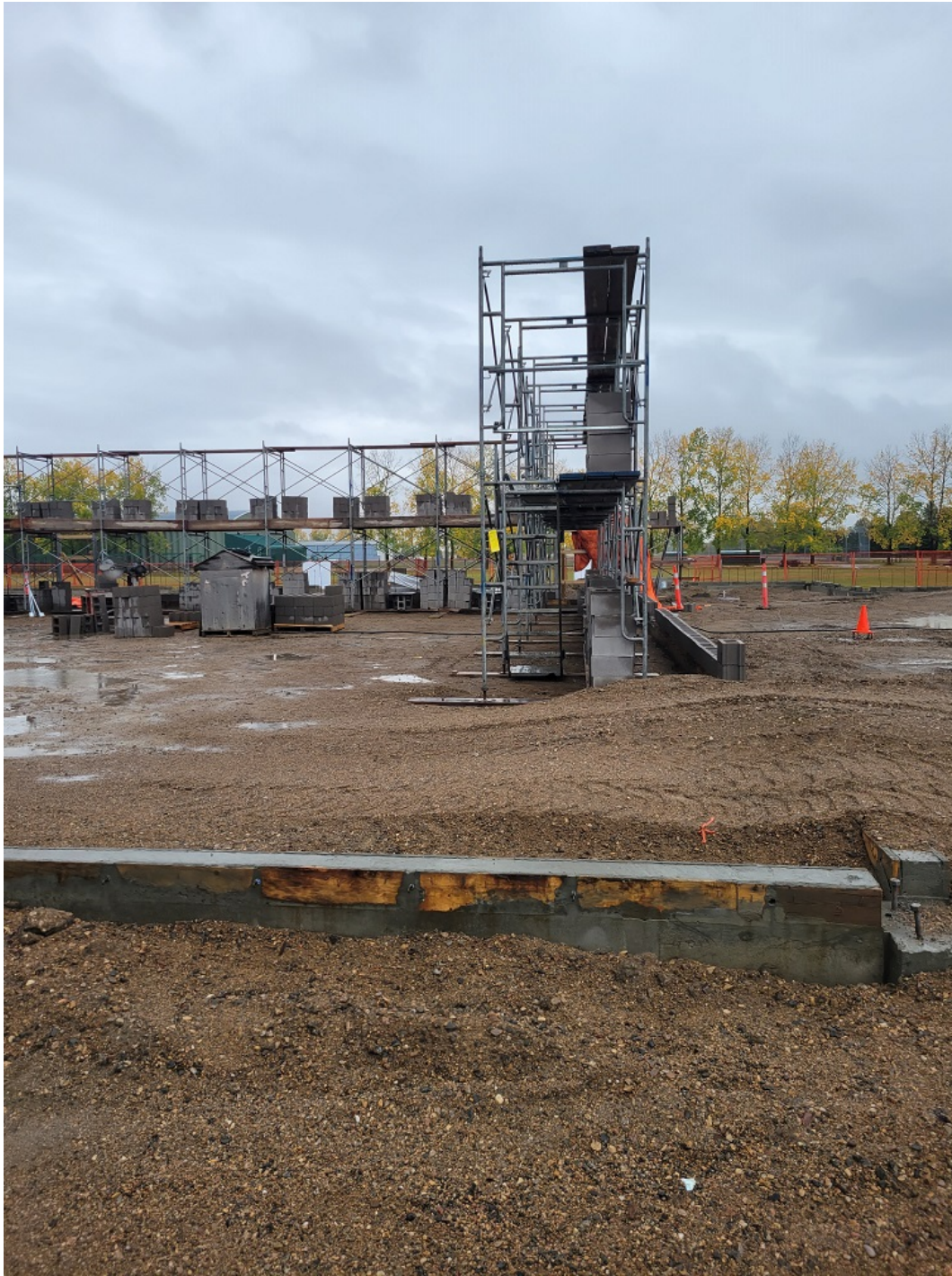
Photo #06 – Room 106 Masonry
