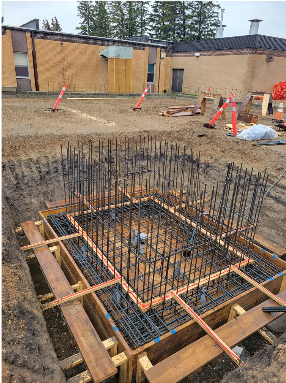
Photo #01 – Elevator Pit
