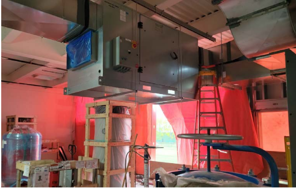
Photo #11 – Mech Room
