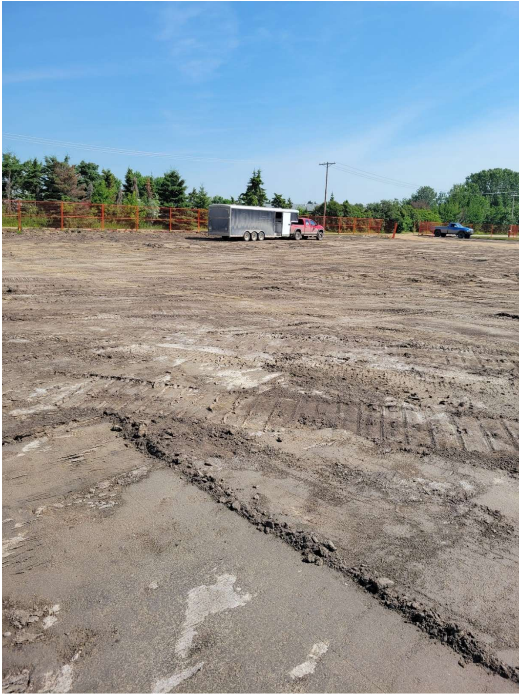
Photo #07 – Stripped Site
