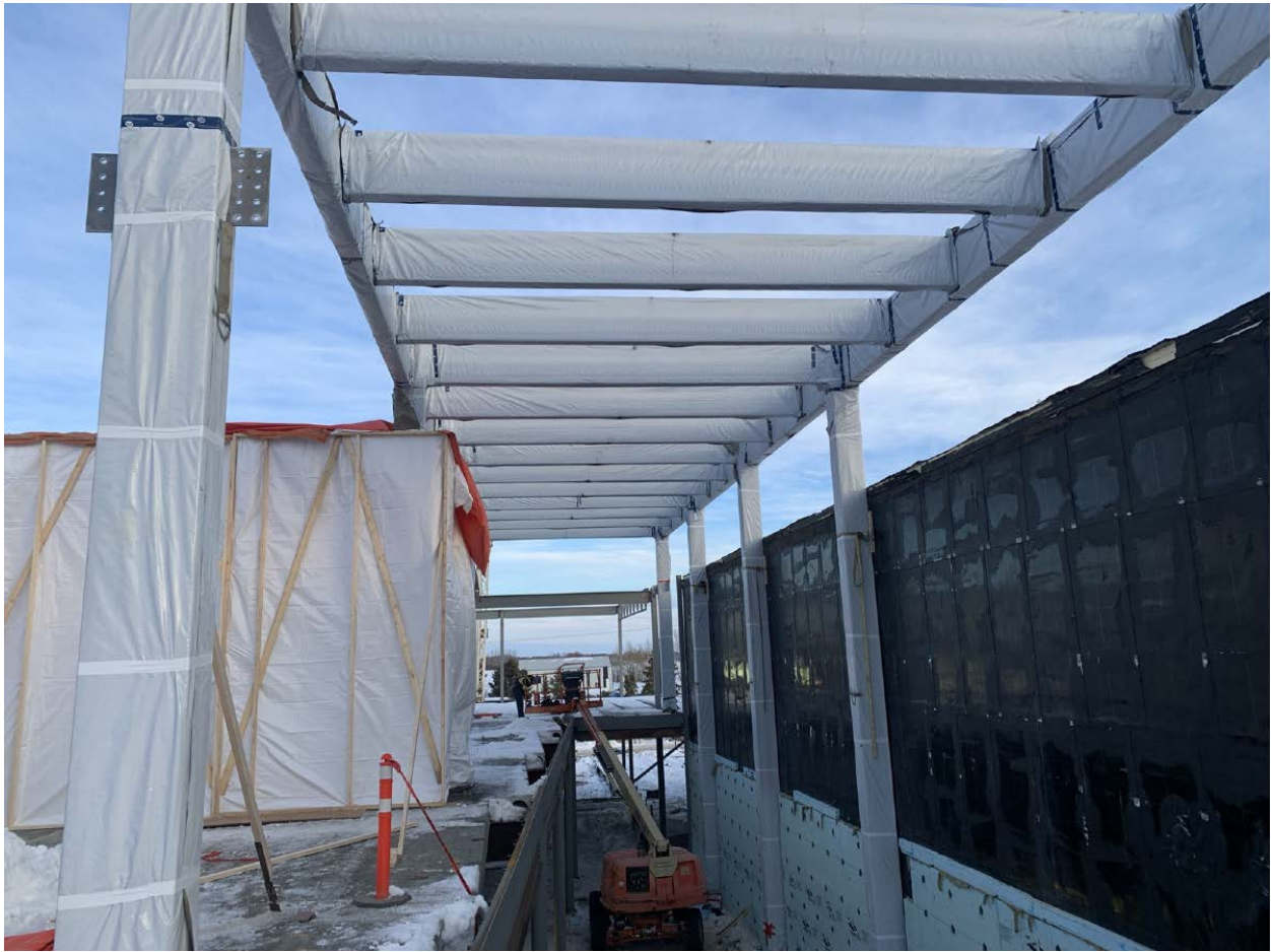
Photo #02 – Glulam installed
