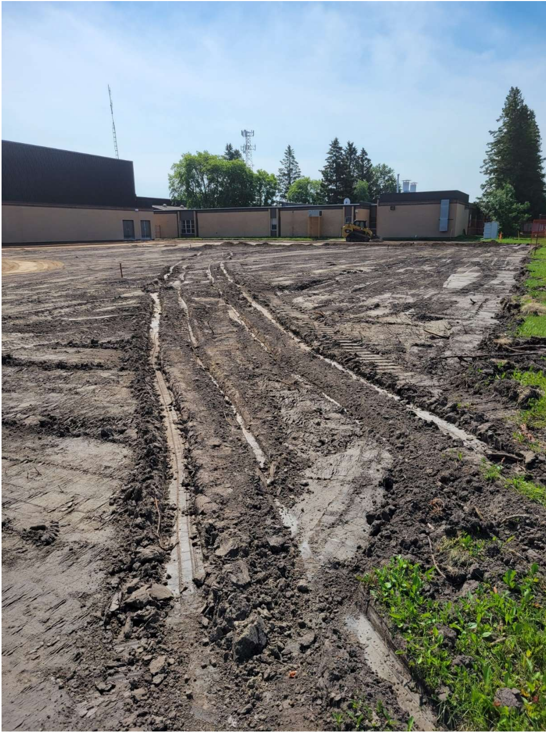
Photo #05 – Stripped Site
