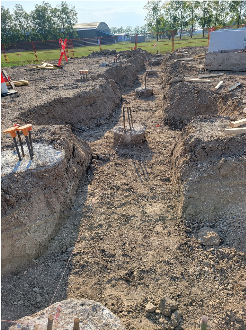
Photo #01 – Piles along Grid Line 3
