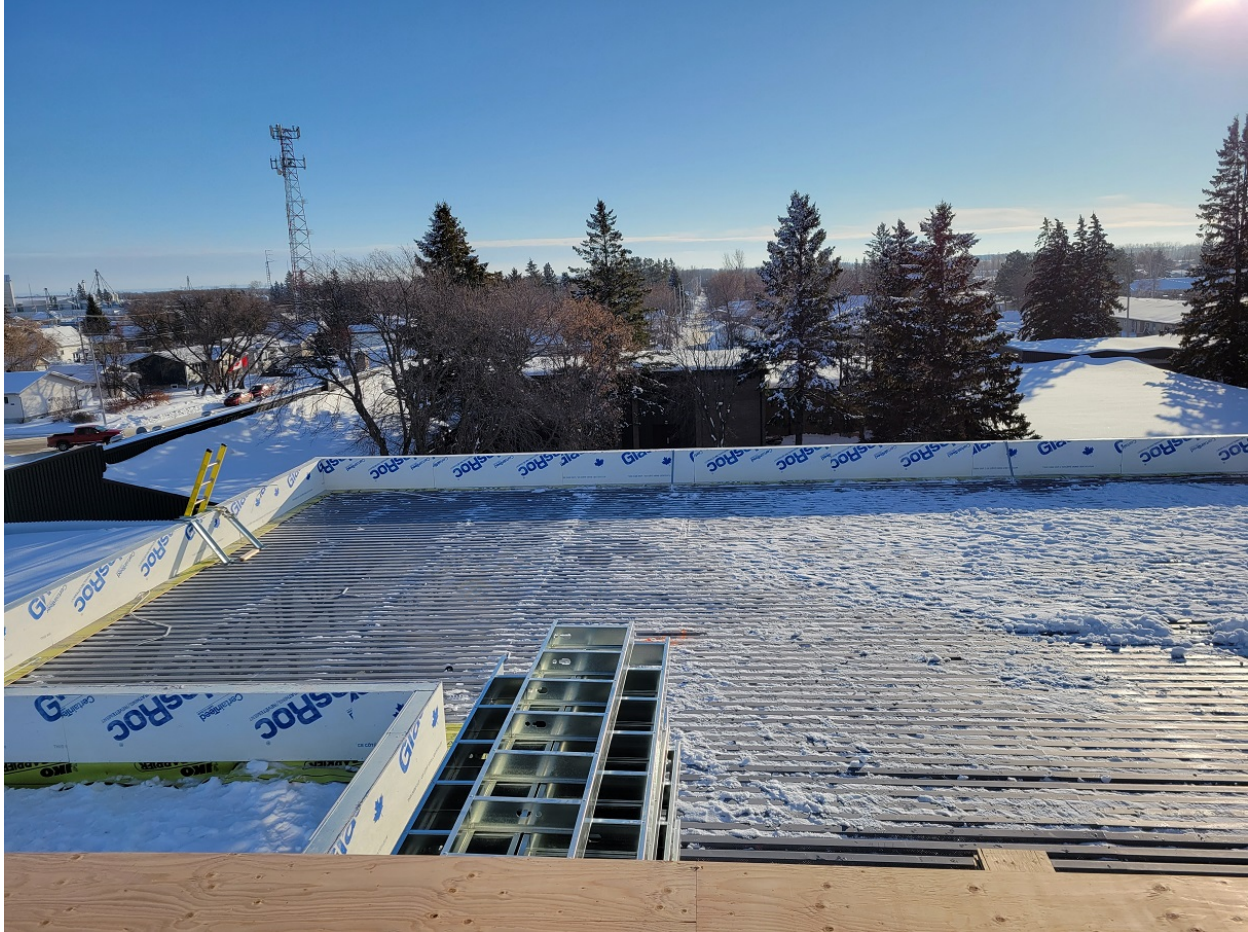
Photo #2 – Roof Parapets over Administration offices
