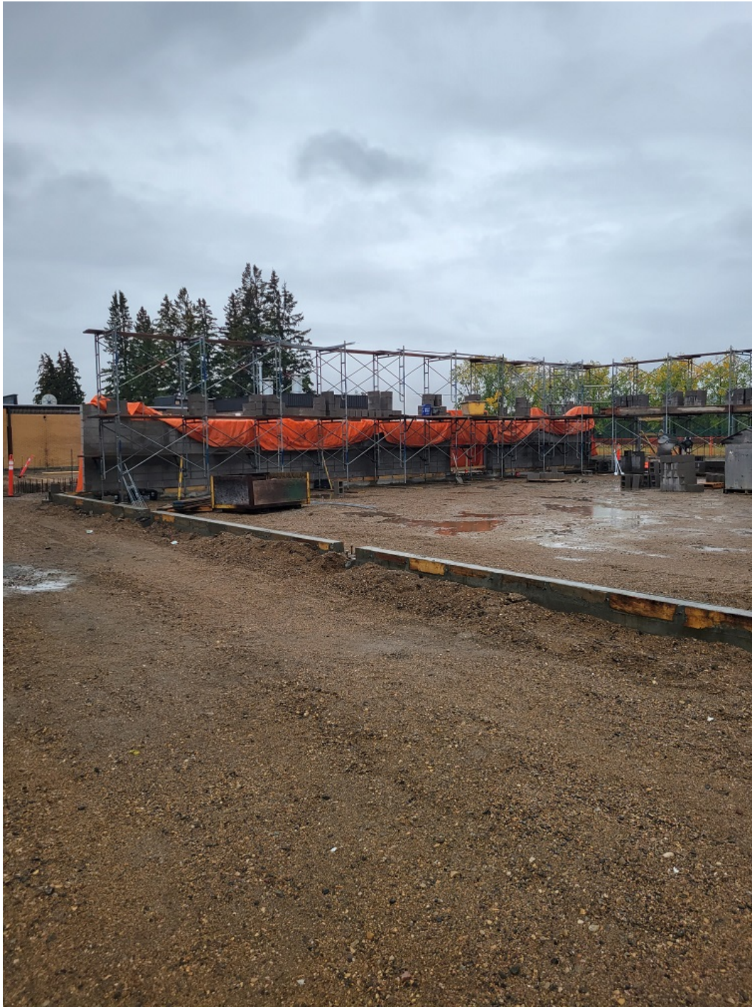
Photo #05 – Room 106 Masonry
