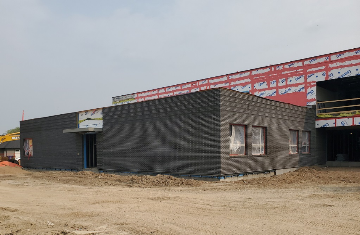
Photo #1 – Exterior Brick on Phase 4
