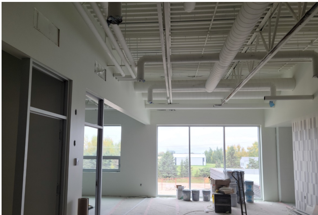
Photo #8 – Corridor 201.2 Flex Rooms Area
