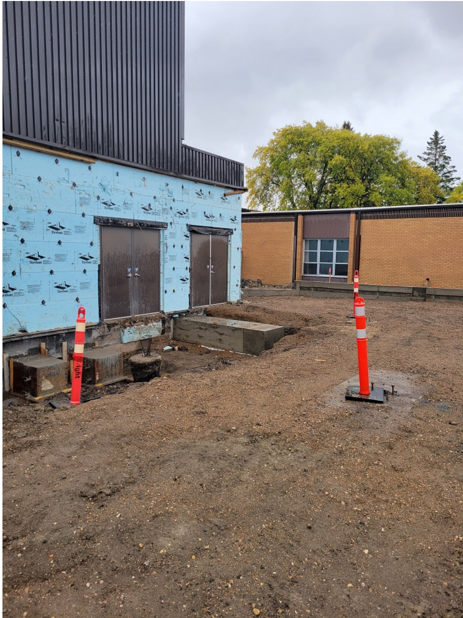
Photo #02 – Front Entrance looking south from Elevator
