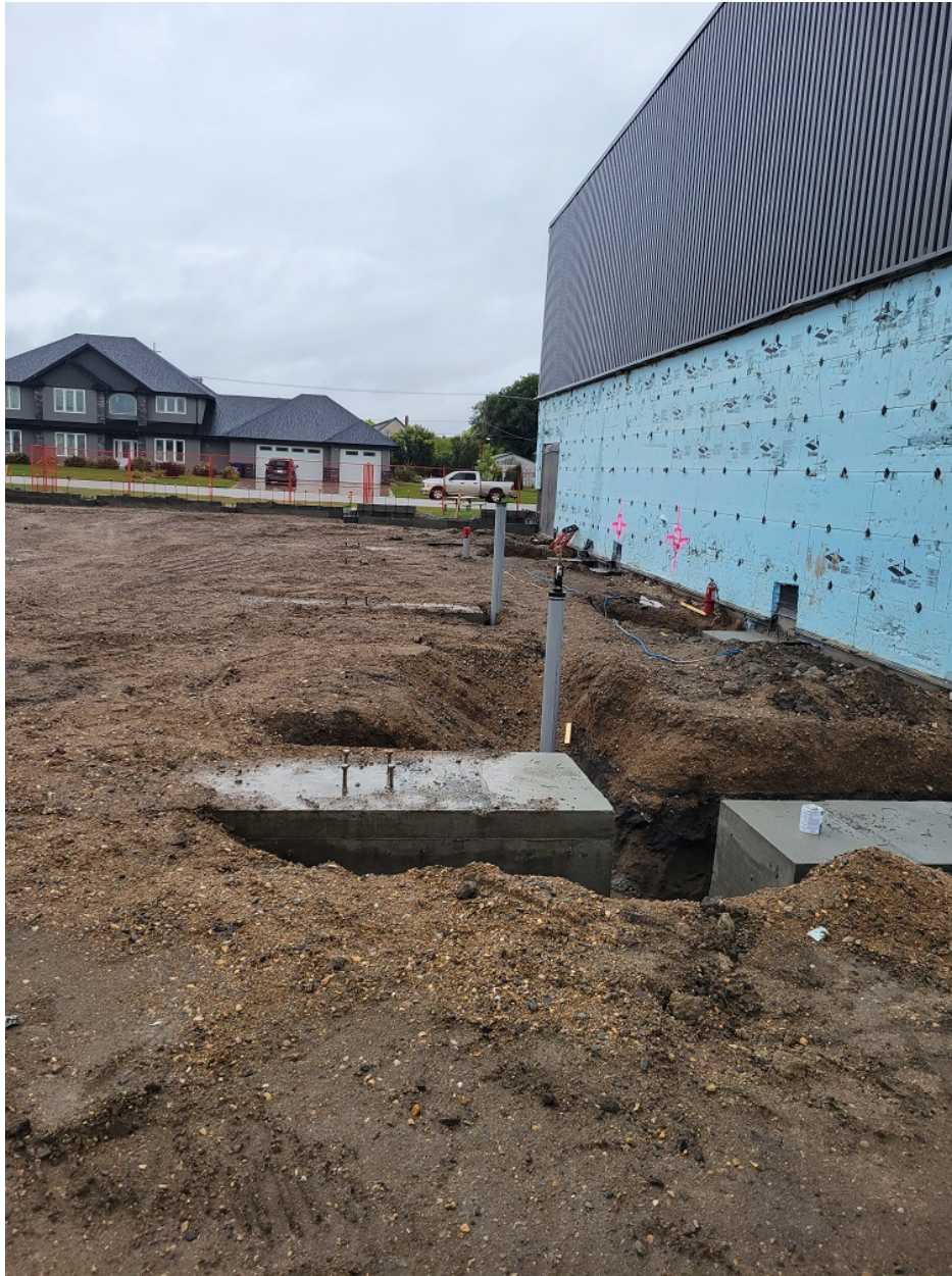
Photo #04 – Piles along Grid Line 5 looking east
