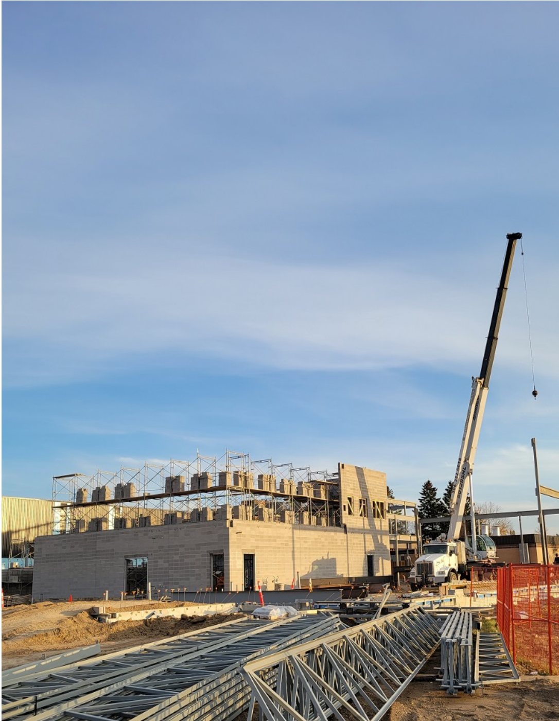
Photo #07 – Room 106 Masonry
