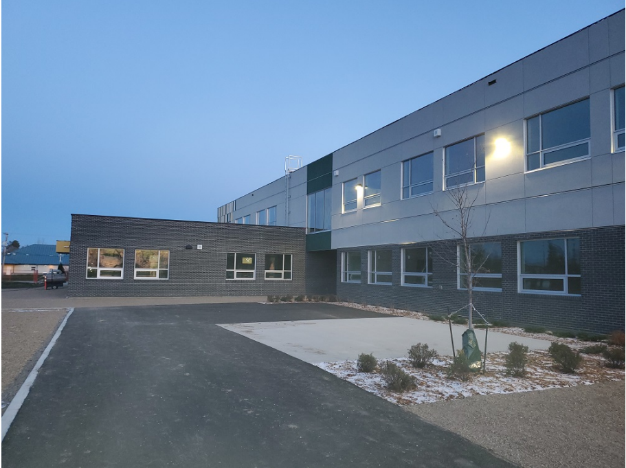
Photo #1 – Site Works
