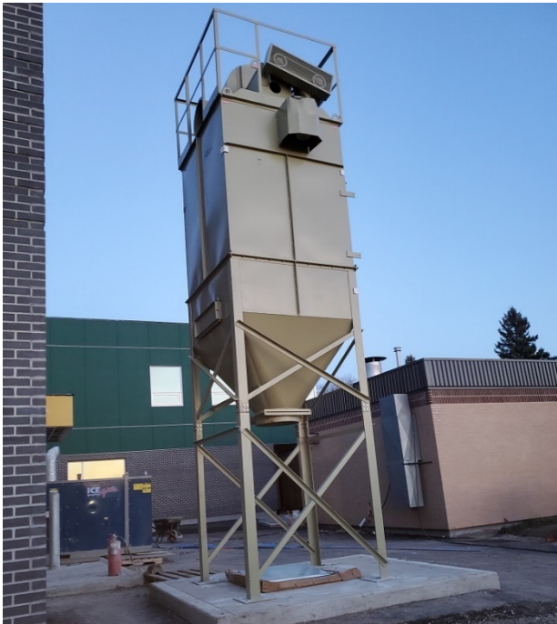
Photo #2 – Dust Collector
