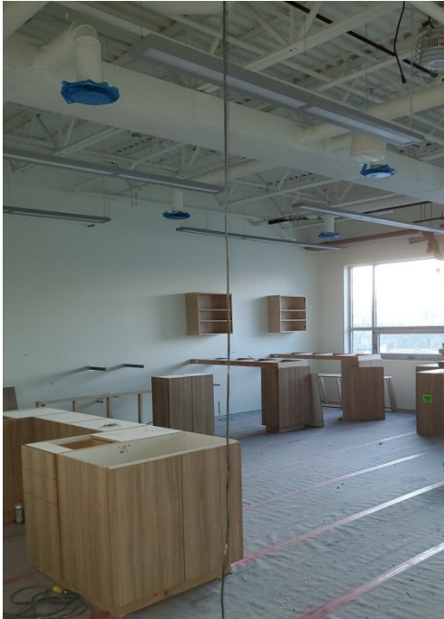
Photo #8 – Science Lab Millwork
