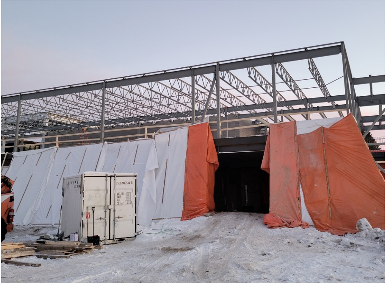
Photo #4 – Hoarding on North West corner
