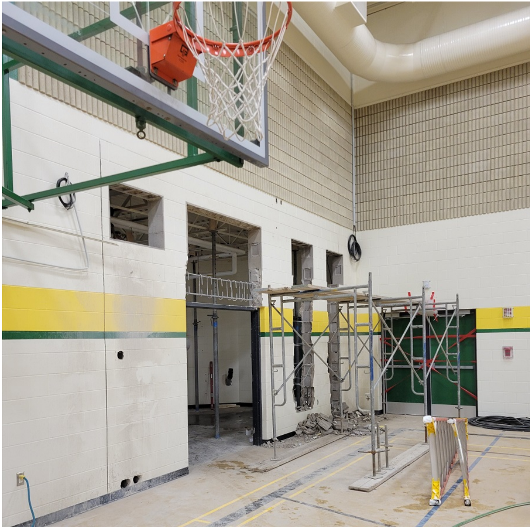
Photo #05 – Existing Gym Storage Demo
