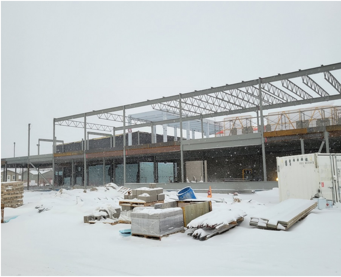
Photo #01 – General site view looking south
