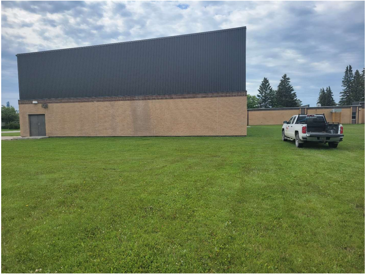
Photo #03 – Pre-Construction, North Side of Gym, Field
