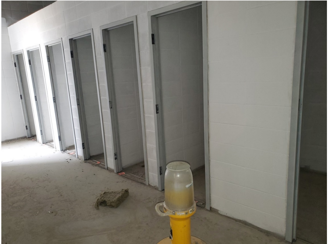
Photo #7 – Second Floor Washroom Block Fill
