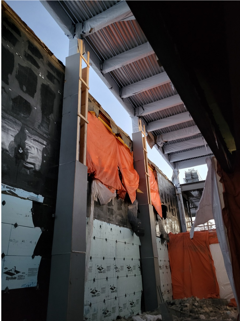
Photo #8 – Clerestory Protection and Roof Deck
