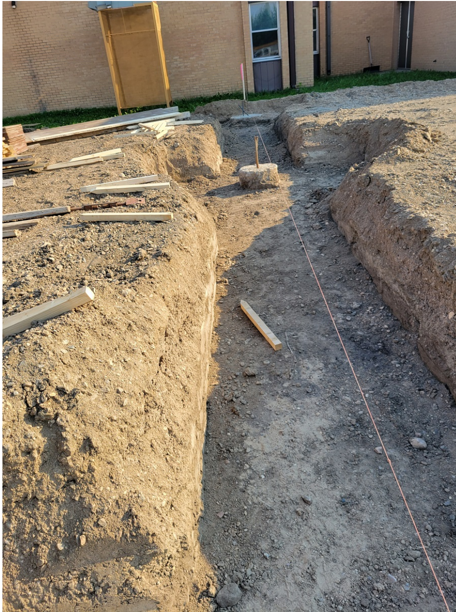
Photo #02 – Piles along Grid Line E looking from Grid Line 5 south
