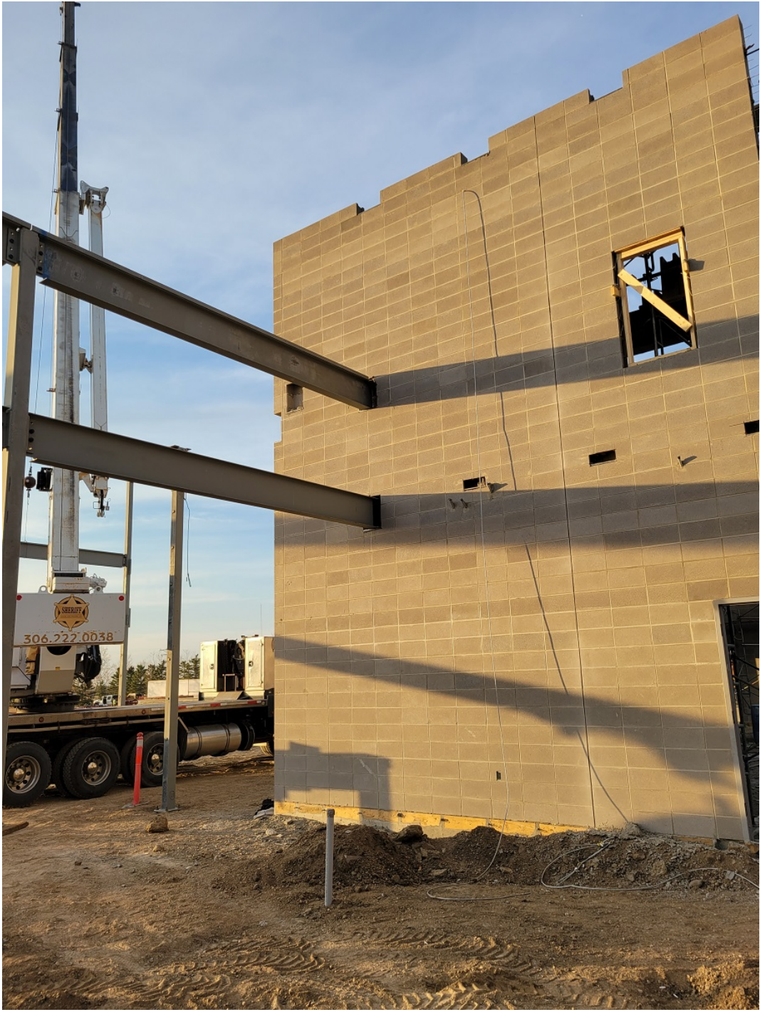
Photo #05 – Room 106 Masonry
