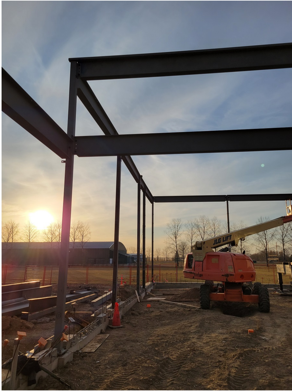
Photo #04 – Structural Steel southwest corner
